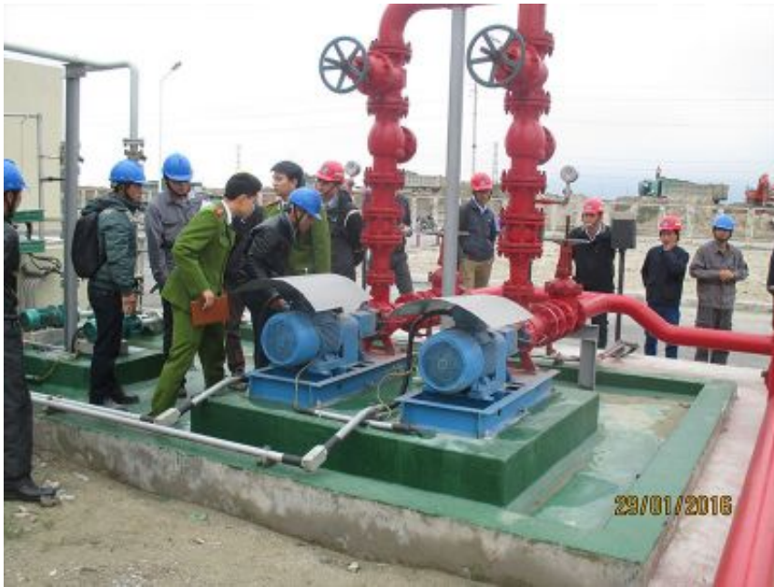
PICTURE OF INSPECTION AND ACCEPTANCE OF FIRE FIGHTING WORKS
