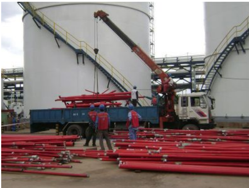
PICTURE OF CONSTRUCTION OF FIRE WATER SUPPLY SYSTEM
