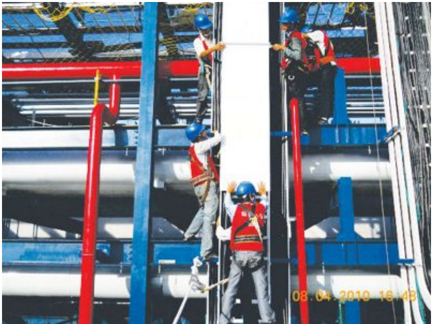
PICTURE OF INSTALLATION OF ELECTRICAL CABLE TRAY - PULLING POWER CABLE
