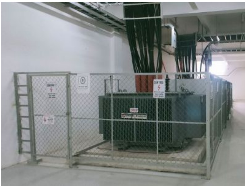
PICTURE OF CONSTRUCTION AND INSTALLATION OF MEDIUM VOLTAGE POWER STATION
