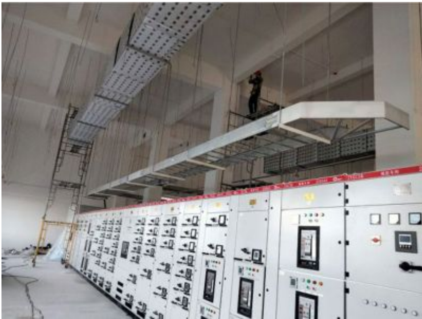
PICTURE OF CONSTRUCTION AND INSTALLATION OF MEDIUM- LOW VOLTAGE ELECTRICAL CABINETS
