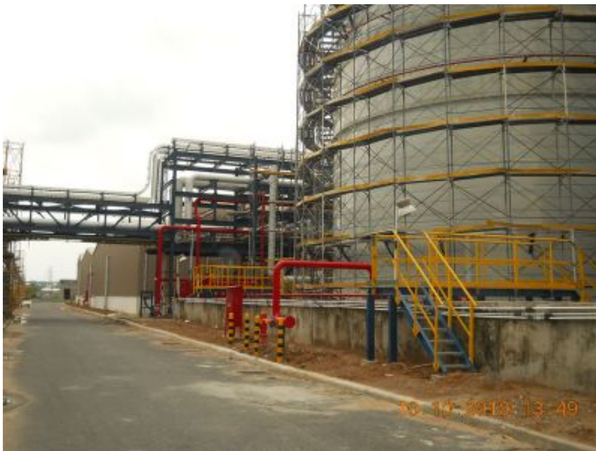
PICTURE OF INSTALLATION OF FIRE WATER SUPPLY PUMP STATION SYSTEM
