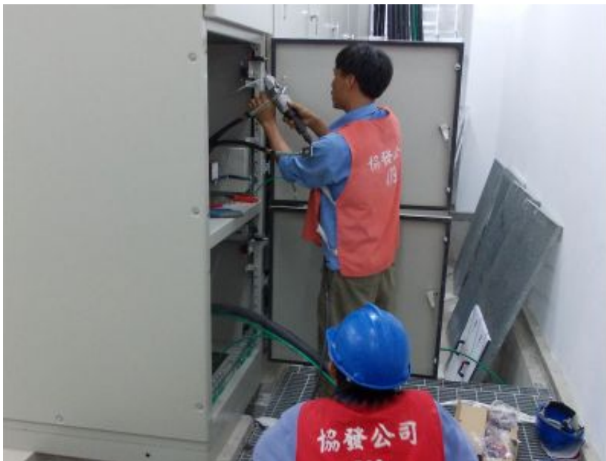
PICTURE OF INSTALLATION OF THE HIGH VOLTAGE CABLE TERMINATION & JOINTS
