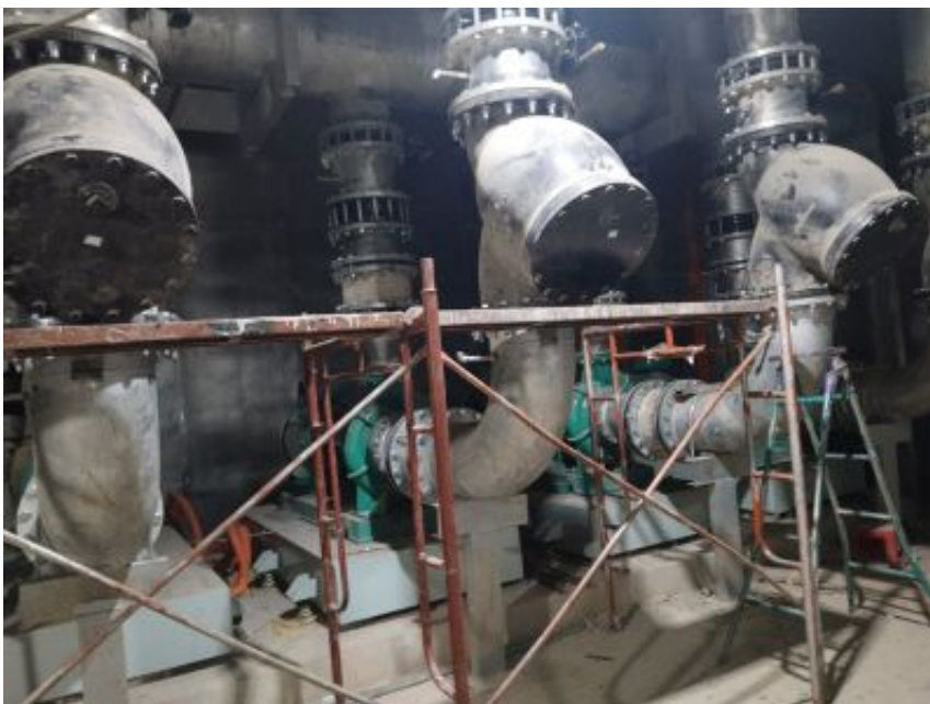
PICTURES OF CONSTRUCTING AND INSTALLING COOLING PUMP STATIONS
