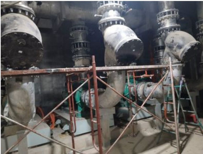
PICTURES OF CONSTRUCTING AND INSTALLING COOLING PUMP STATIONS
