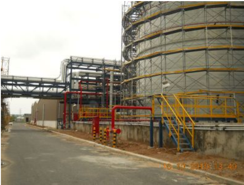
PICTURE OF INSTALLATION OF FIRE WATER SUPPLY PUMP STATION SYSTEM
