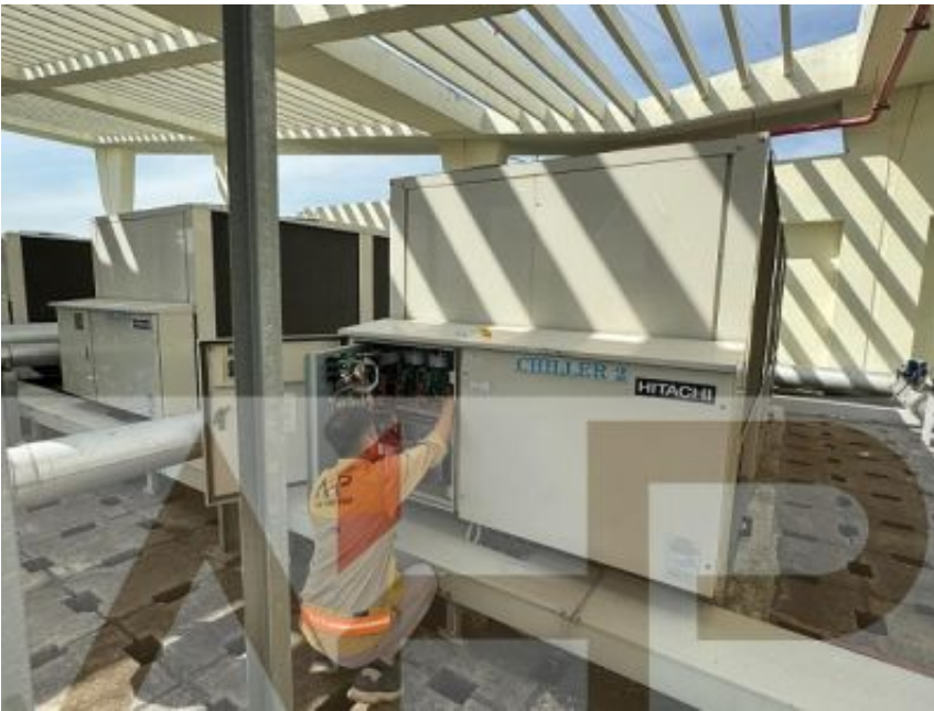
INSTALLATION OF CHILLER SYSTEM IN OFFICE BUILDING
