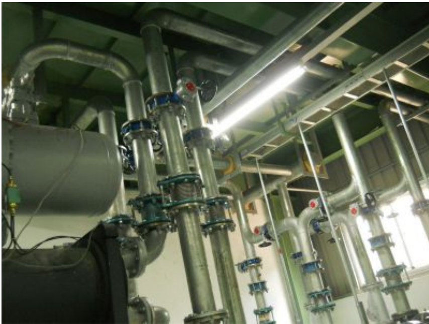
PICTURES OF CONSTRUCTING AND INSTALLING CHILER COOLING MACHINES
