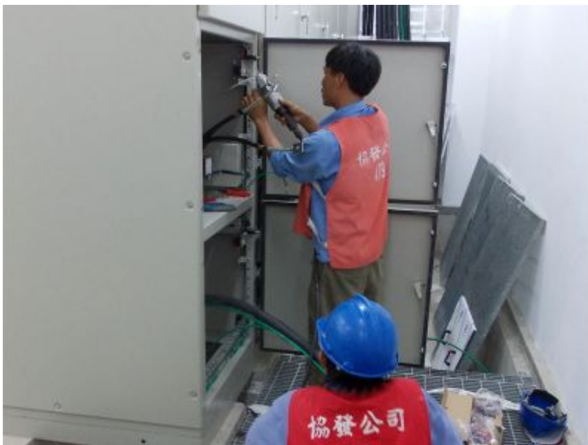
PICTURE OF INSTALLATION OF THE HIGH VOLTAGE CABLE TERMINATION & JOINTS
