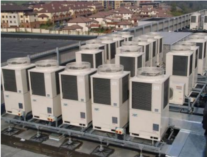
PICTURES OF CONSTRUCTING AND INSTALLING VRV CENTRAL REFRIGERATION SYSTEMS
