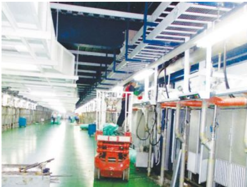
PICTURE OF INSTALLATION OF THE FACTORY LIGHTING SYSTEM
